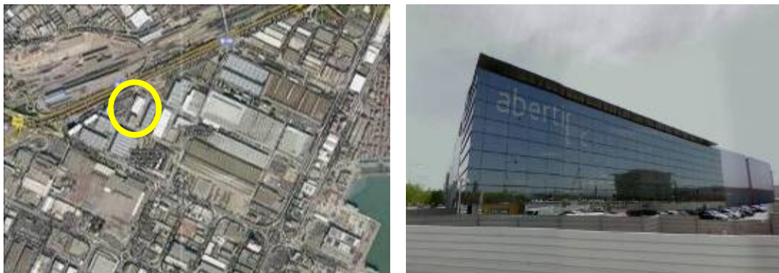
Figure 2.5.2. Abertis facilities top view (left) and front view (right)
